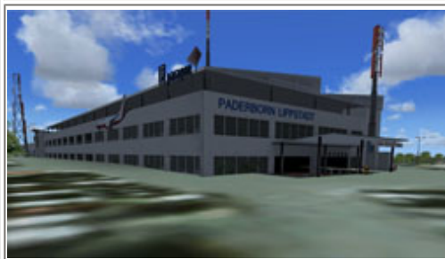
Again another example of good building models but the surrounding areas such as roads, etc may have deserved a little more attention
